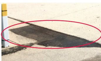
Pavement: Elevation Change Repaired
