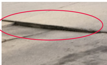
Pavement: Elevation Change Repaired
