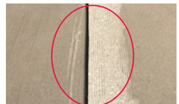
Pavement: ground to remove higher edge to remove trip hazard.
